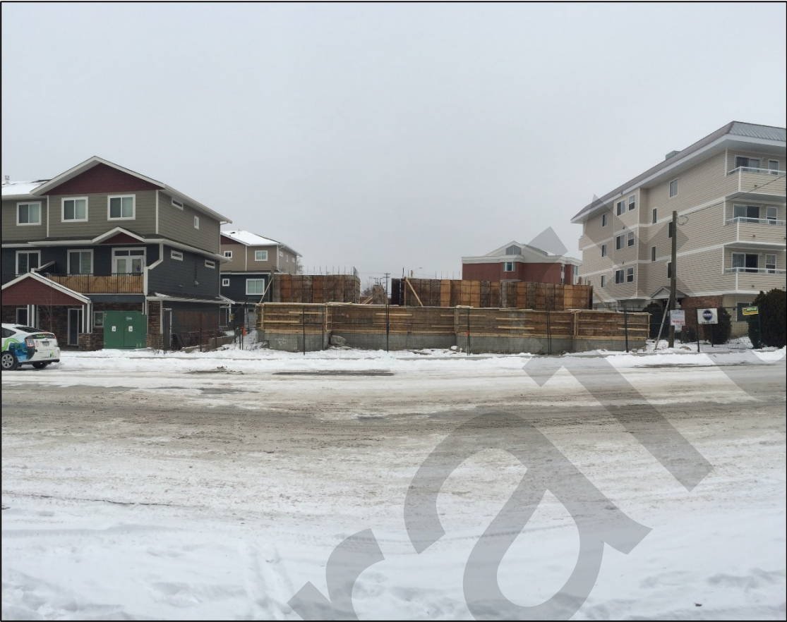
Figure 4: South View of Subject Property
